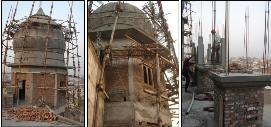
Figure 6.83: Masonry Dome under construction, scaffolding around dome for finishing and carving details and the base of the chhatri along with 4-6 columns is at initial stage for the construction
