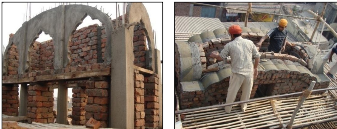
Figure 6.84: Chhatri Under construction
