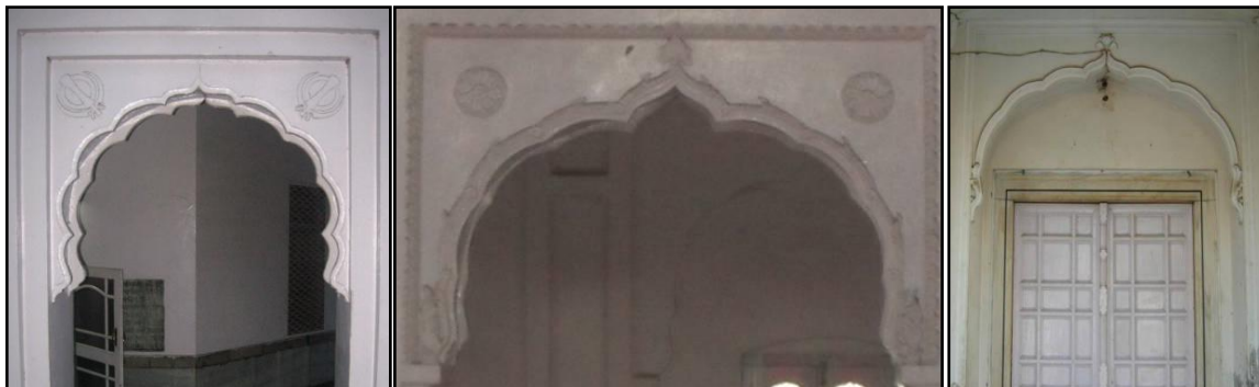
Figure 6.74: Cusped Arches in the Sikh Shrines
